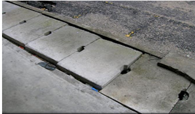
Figure 3. Concrete drain cover
