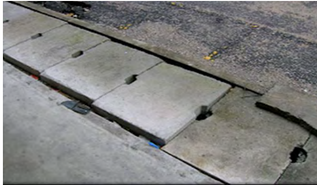
Figure 3. Concrete drain cover
